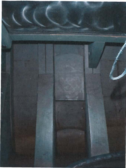
Properly installed beveled and radiused butt blocks
