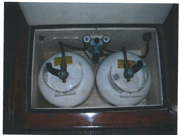
ABYC compliant propane locker
